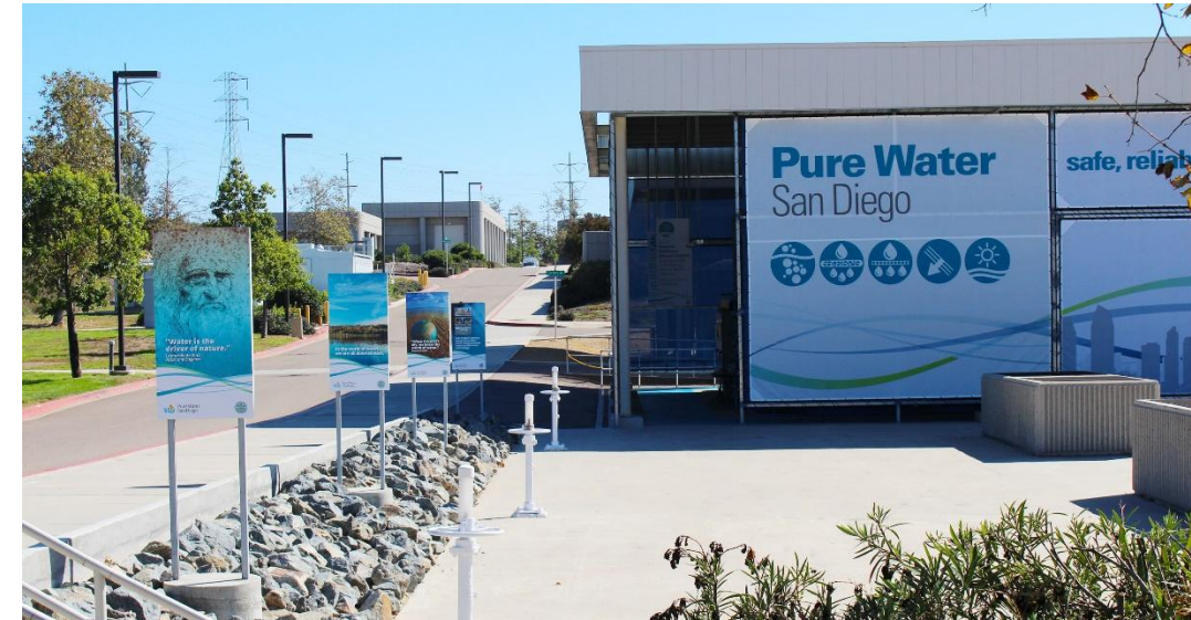
Pure Water San Diego Demonstration Facility
